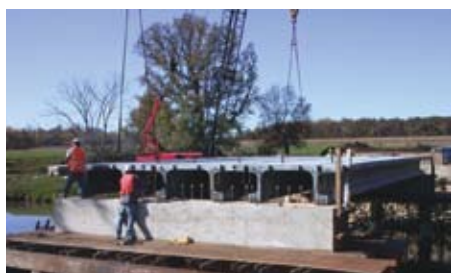
Pont Jakway Park Iowa (Etat-Unis)
